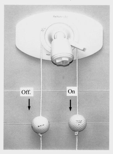
**6/.** Extend the braided cord down and adjust the knots below the two balls to a height that suits. Now when you pull down on the right hand ball the shower turns on, pull on the left one and the shower turns off.
