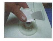
9/. Slide on the remote lever until it sits hard against the wheel . N B both the remote lever and the shower lever should have the same angle of position. See drawing opposite
