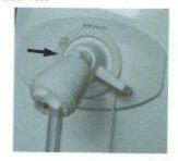
5/. Replace the rose by screwing in clockwise.
